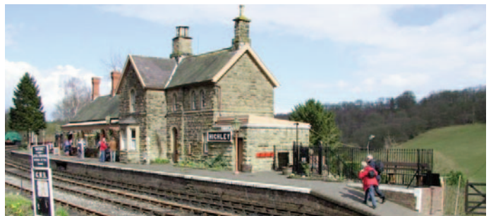
Highley signal box and Highley station.
